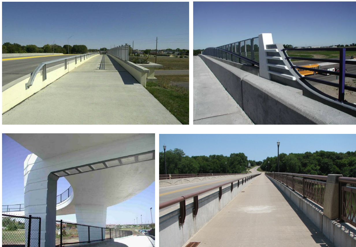
Figure 9.5.3.11. Example of handling aesthetics on a bridge widening
