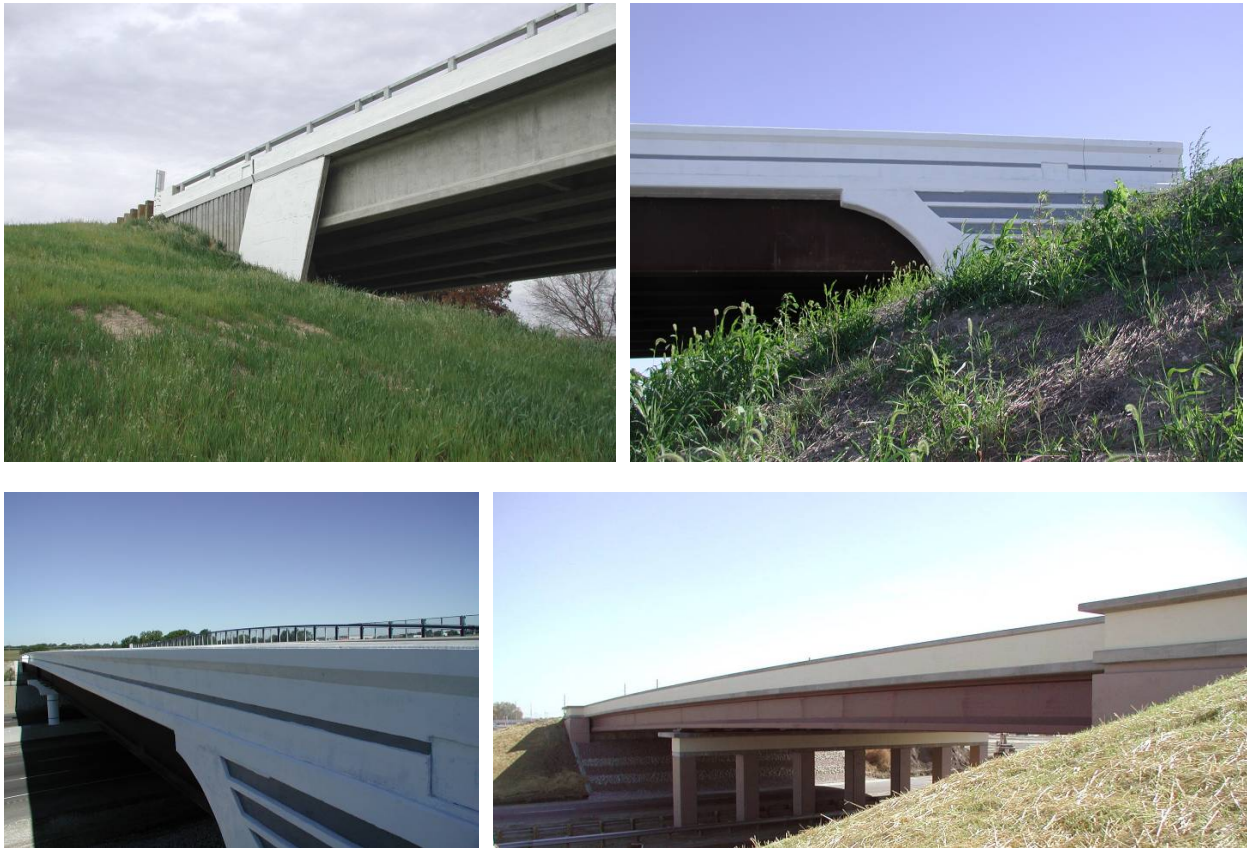
Figure 9.5.3.1. Bridges with long, slender appearance
