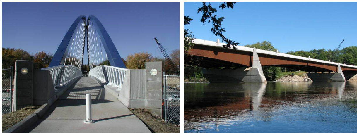
Figure 9.4.4. Level “A” bridge examples in Iowa
