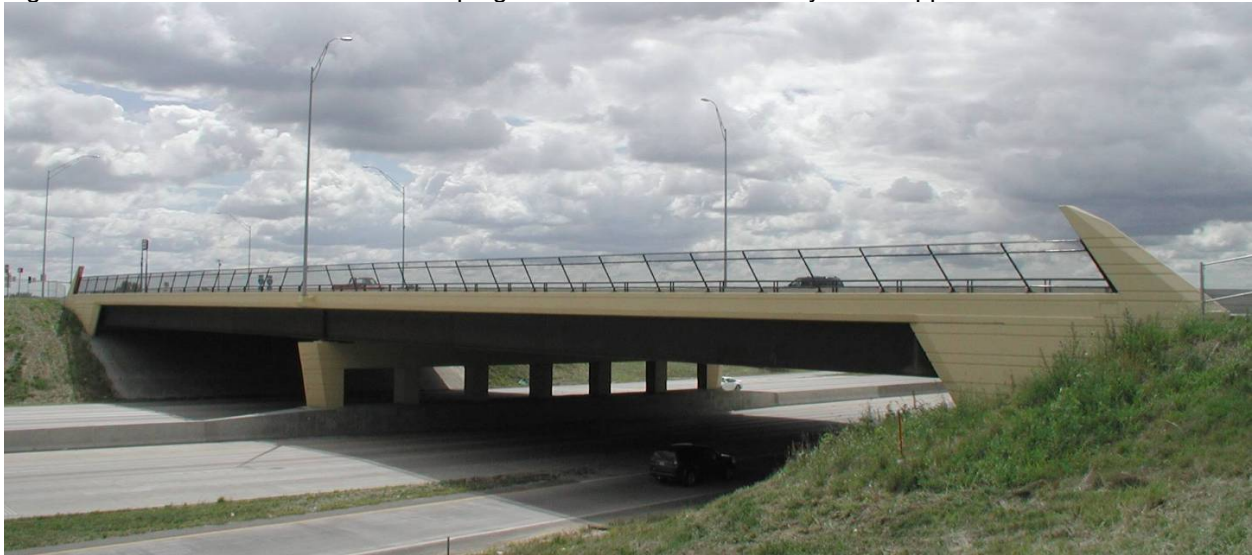
Figure 9.5.3.6. Bridge with sloping mask wall
