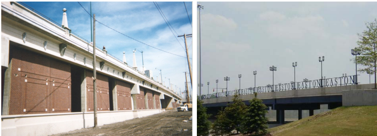
Figure 9.5.3.7-1. Bridges with ineffective bolt-on aesthetic details
