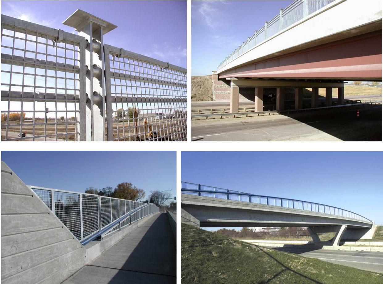
Figure 9.5.3.7-2. Bridges with complementary bolt-on aesthetic details
