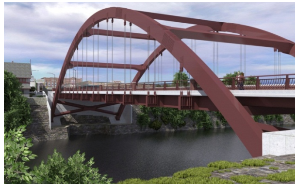
Figure 2.3.1-2 Replacement Steel Arch Bridge
